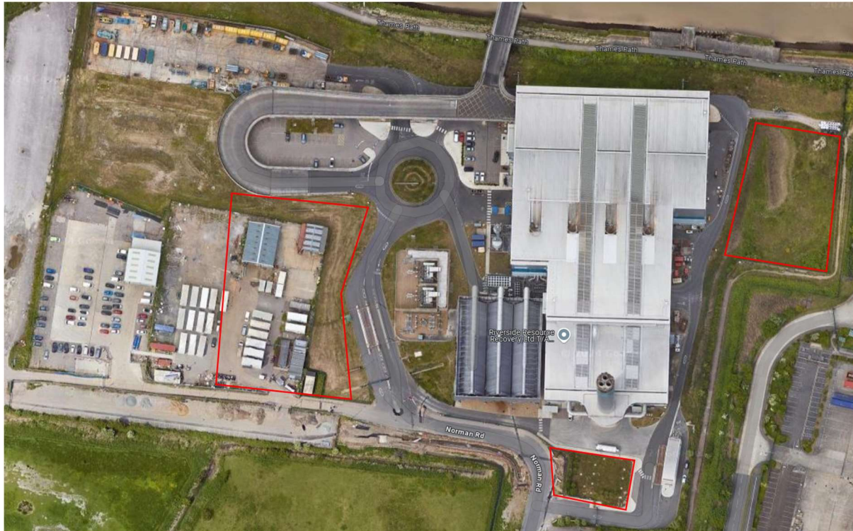
Figure 7- Apparently unutilised space on Riverside 1 EfW
